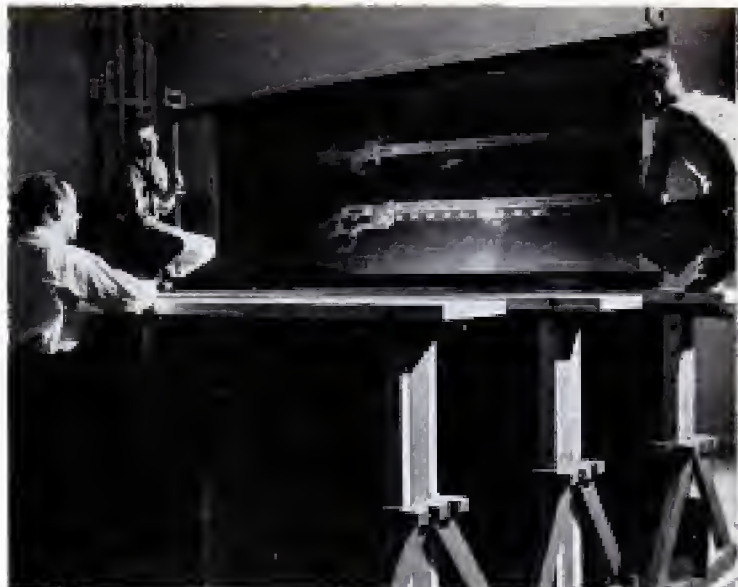
Rifles are suspended between betatron, top left, and film platform, below. Right, finished X-ray picture
